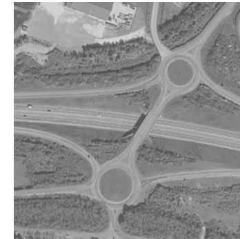
Scotland Road dumbbell junction
