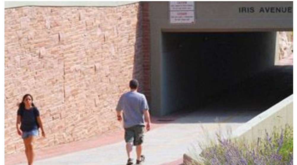
Culvert © Boulder-Buzz (cc-by-sa/2.0)
