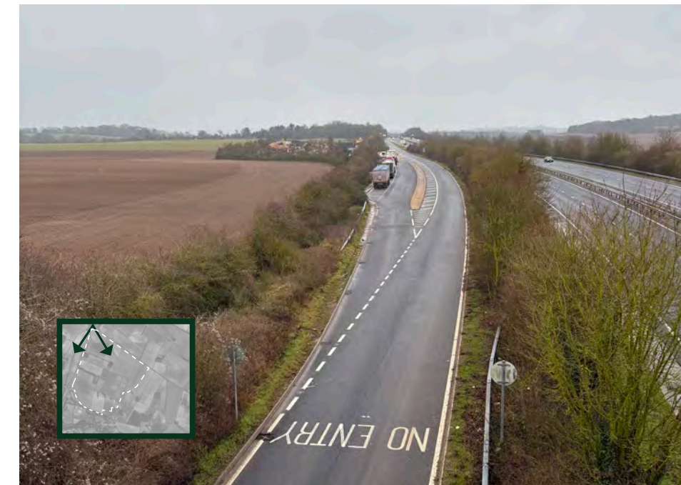
Slip road off A11
