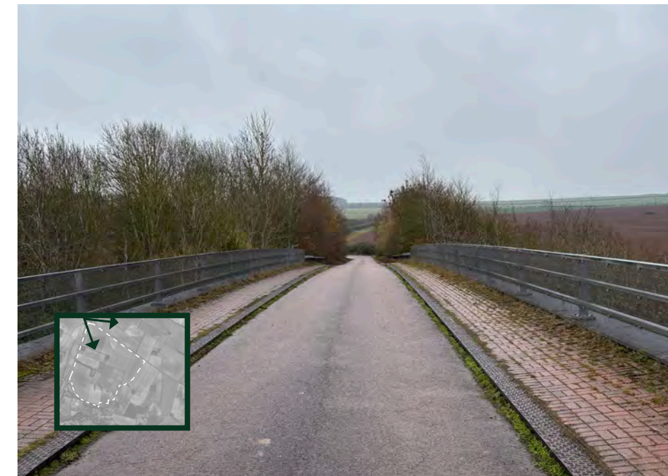
Bridge over A11
