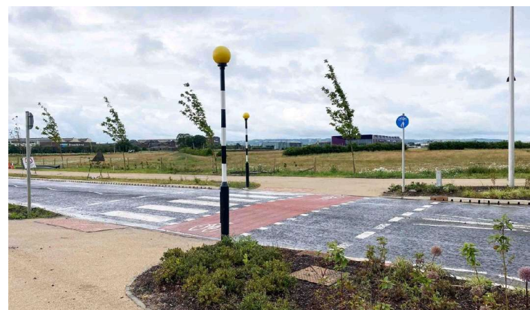
Figure 32: Example of Parallel Crossing installation
