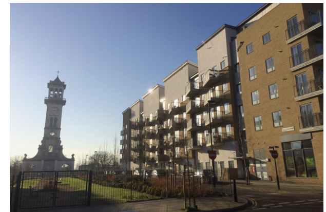
Image 13: North Road Estate Renewal - successful regeneration project providing street blocks of coherent height that enhance the setting of the historic clock tower (Camden, London)
