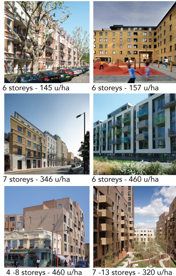
Figure 7: Comparison of residential density (units per hectare) across developments of different heights (Housing Density Study, Maccreeanor Lavington, 2012)
