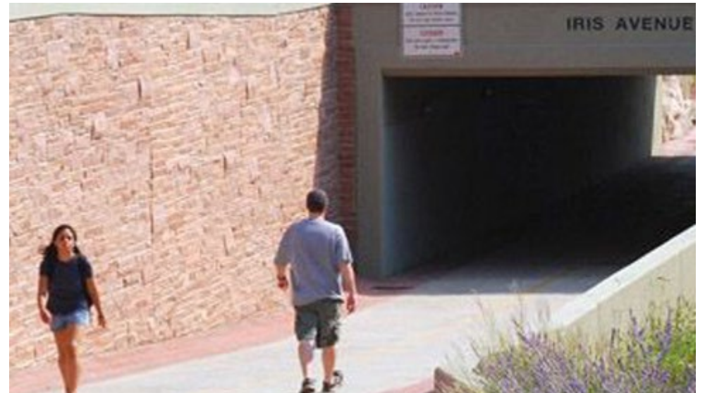
Culvert © Boulder-Buzz (cc-by-sa/2.0)
