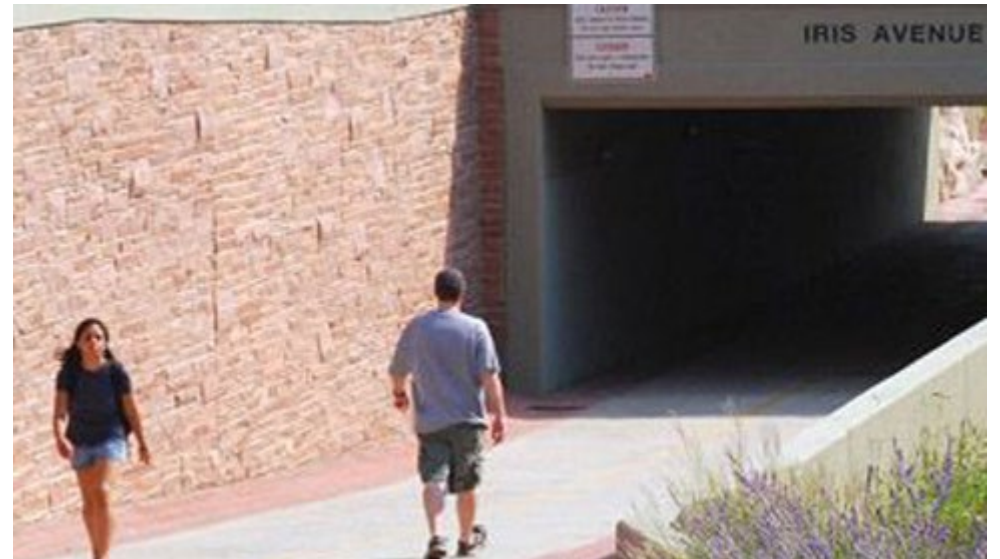
Culvert © Boulder-Buzz (cc-by-sa/2.0)
