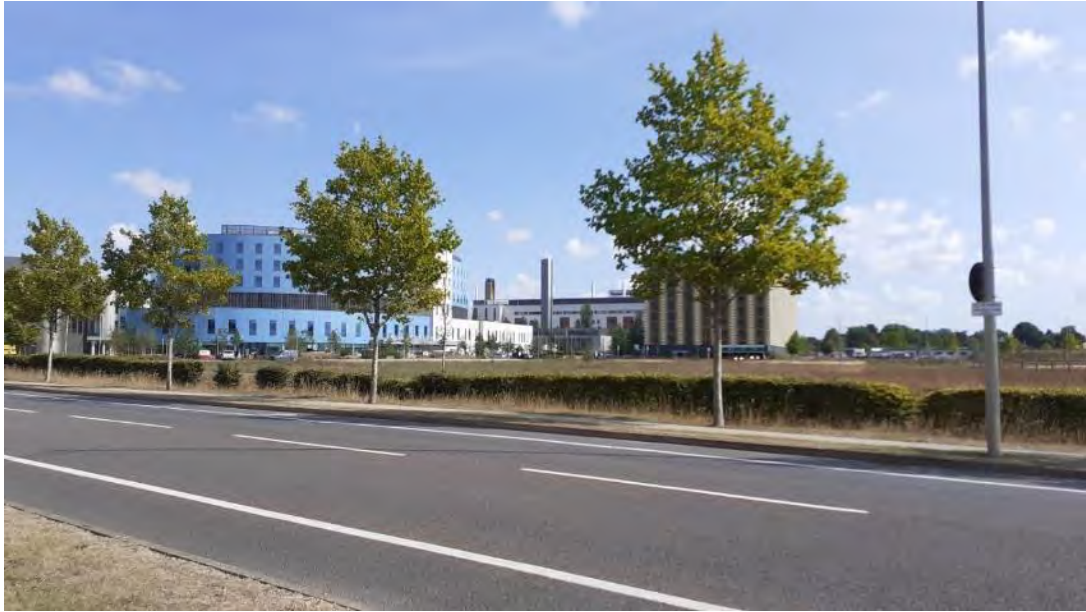
Plate 5. View of hospital buildings in the north of the study site, facing north-east
