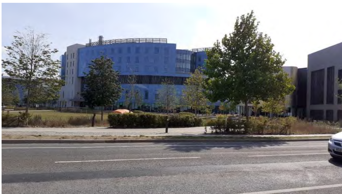
Plate 4. View of the Royal Papworth Hospital in the west of the study site, facing east
