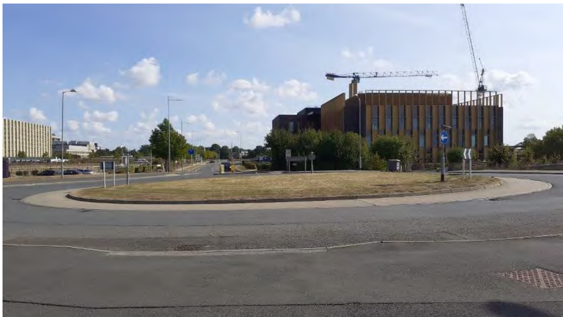
Plate 8. View of the AbCam building from west of the study site, facing eastwards
