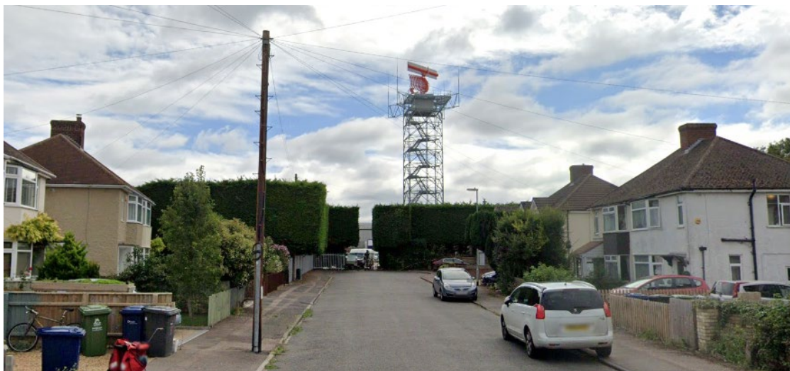
Figure 7.5: Airport radar tower rising above Barnwell residential properties
