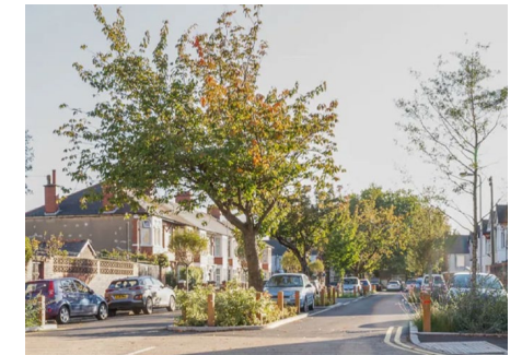
108 rain gardens added to streets in Grangetown, Cardiff, providing storage of 40,000m 3 (40,000,000 litres) of surface water ( Link )
