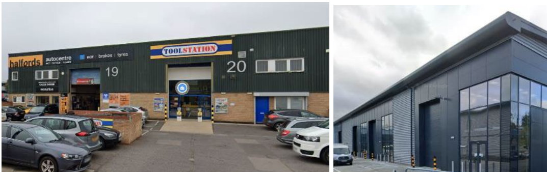
Figure 2.1 Industrial Units – Clifton Road, Cambridge / Bar Hill
