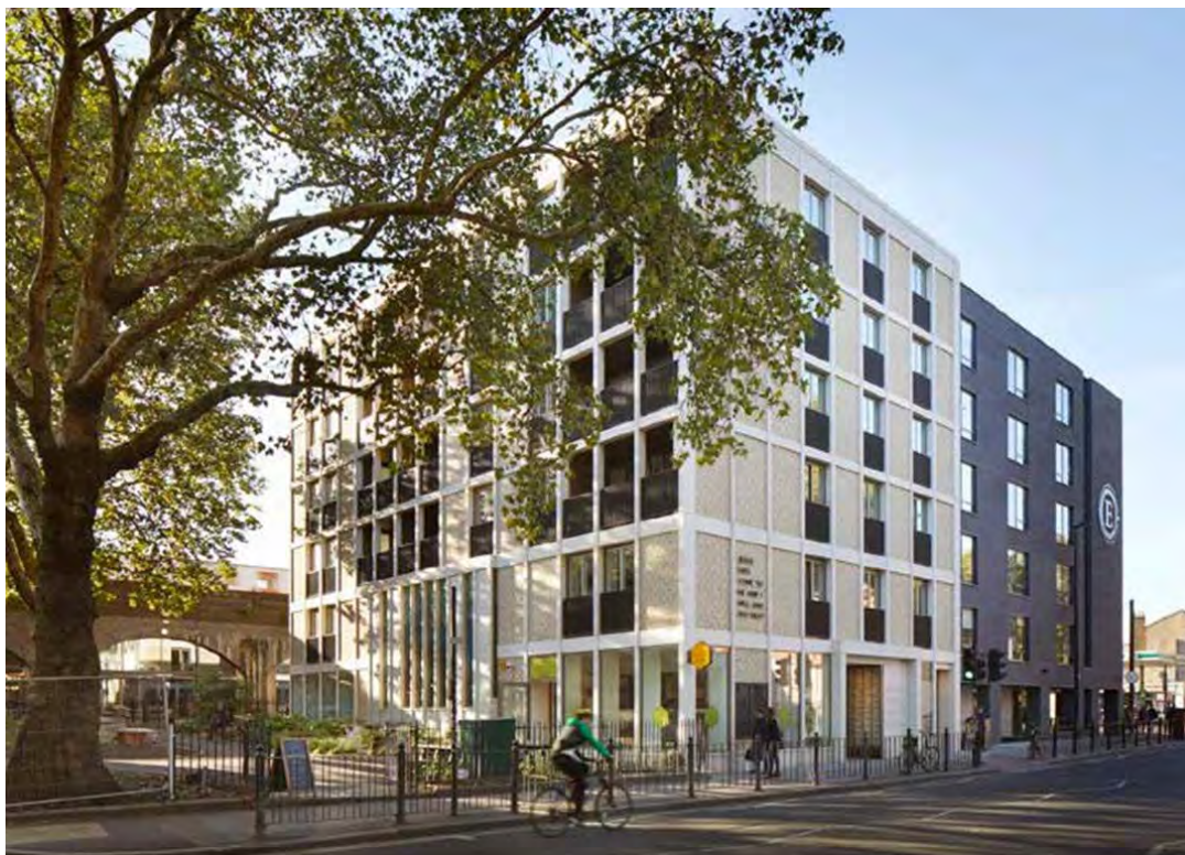
Image credit: Gatti Routh Rhodes Architects and Jack Hobhouse
